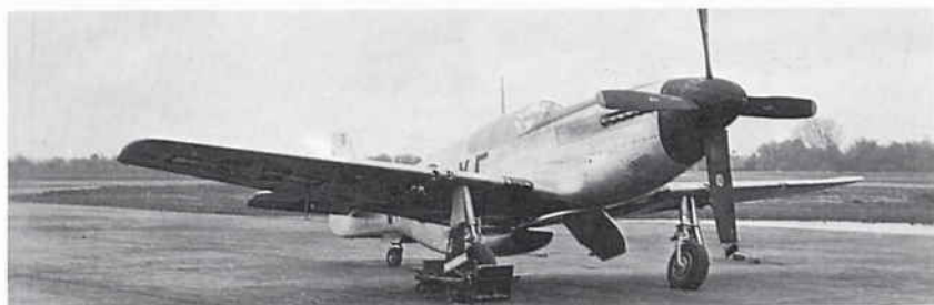
Below: P-51B, 4th FG, 336th FS, in natural metal finish with red spinner and nose after heavy landing at Debden. Note undercarriage somewhat bent. a/c letter V. (Ray E. Bowers).
