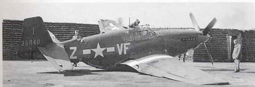
Below: P-51B, 4th FG, 336th FS, in natural metal finish with red spinner and nose after heavy landing at Debden. Note undercarriage somewhat bent. a/c letter V. (Ray E. Bowers).
