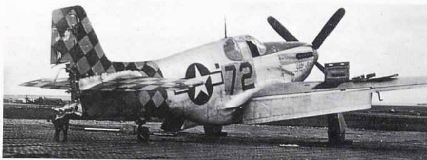
'Lady Jean' with half its rudder shot away, probably by flak, made it back to Lesina safely. 325th Fighter Group, 15th Air Force, Italy. (via E. R. McDowell).
