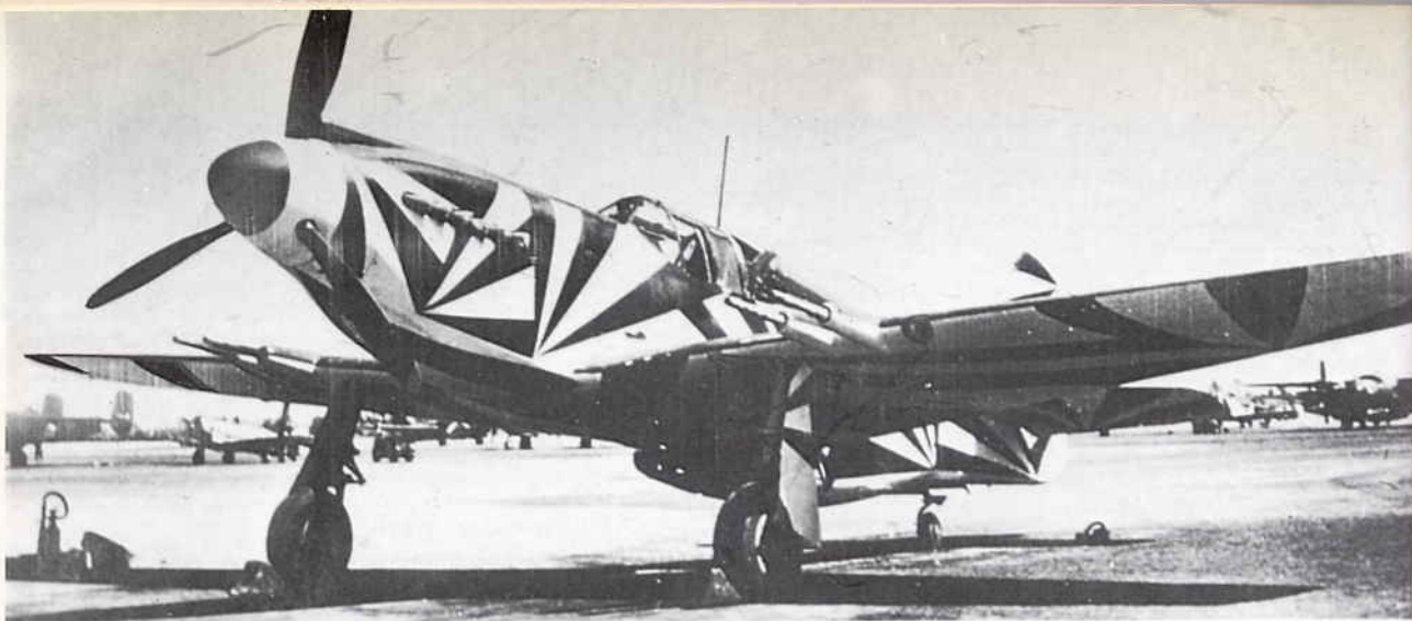
P-51 modified for photo recon duties with camera aft of cockpit in experimental camouflage scheme. See colour illustration. (photos USAF).
